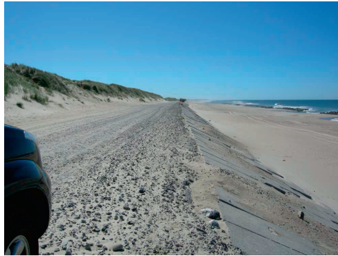
Figure 5.14: Dune with revetments near Thorsminde, along the North Sea coast of Denmark
